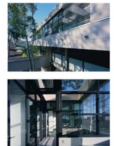
Connecting indoor and outdoor spaces.
