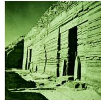
Wall revealing soil strata
